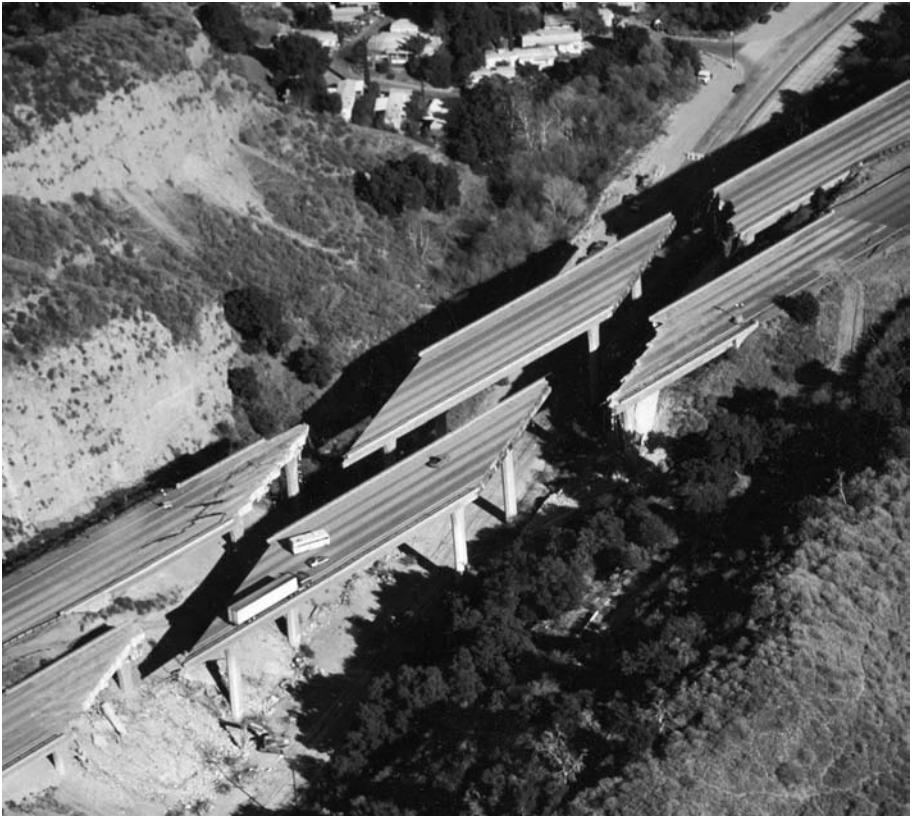
Figure 1.1 “Natural” disaster. In this area earthquakes are natural and frequent, while the “disaster” resulted from a bridge in this location which was unable to withstand the earthquake. Gavin Canyon, Los Angeles County, California; earthquake 6.8 on Richter scale. The absence of housing on these slopes near Los Angeles prevented worse effects. Photo courtesy of US Federal Highway Administration.
