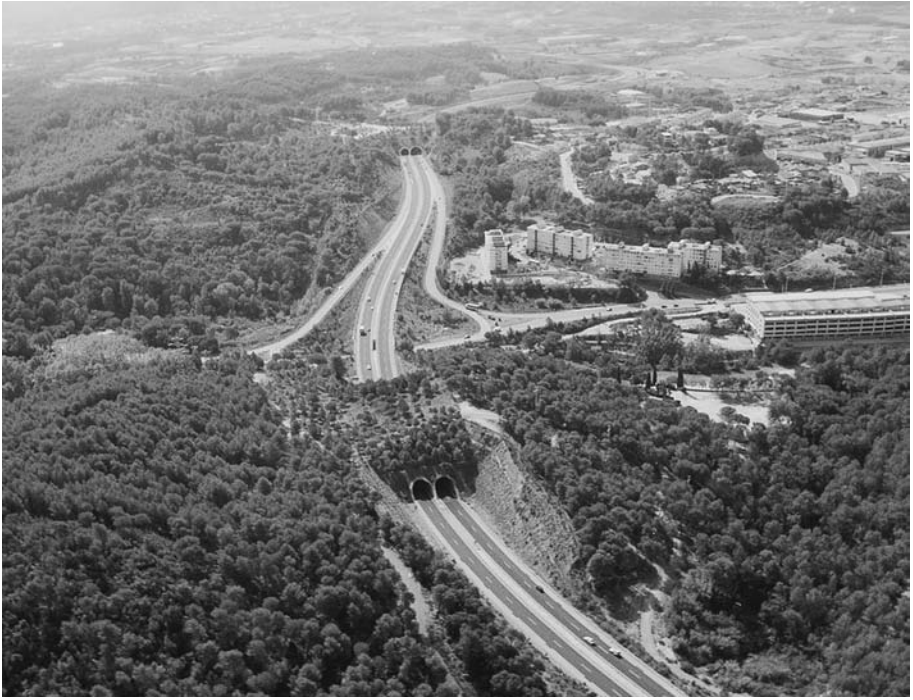
Figure 11.2 Two vegetation-covered overpasses across a multilane highway. Only 12 km from center city Barcelona, these provide connectivity for local residents, hikers, and wildlife, and were built when the Ministry of Environment concluded that a new highway should not disrupt connectivity of the landscape. Carretera de los tuneles. R. Forman photo courtesy of Josep Acebillo and Marc Montlleo.
